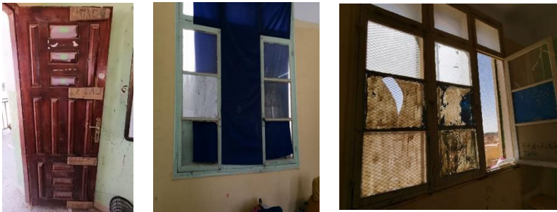
Fig 2. The Windows and Doors in the Middle School
