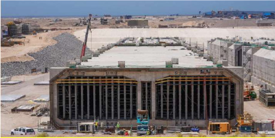
Figure 1: Pouring one of the canal sections submerged in the canal, 2024. Source: Ports Magazine, State Directorate of Iraqi Ports, 65 th year, No. 466, 7.
